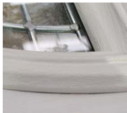
Over-tight. Deformation
